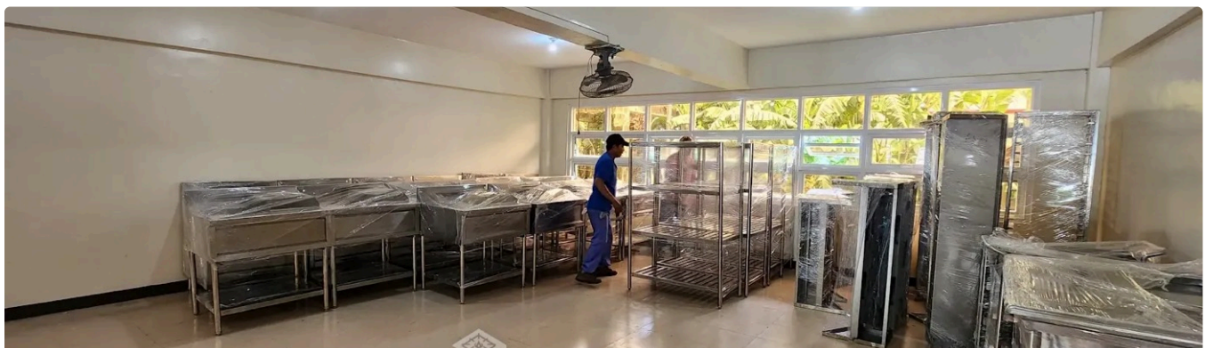
DMMMSU: room installed with stainless-steel tables, racks and shelving
