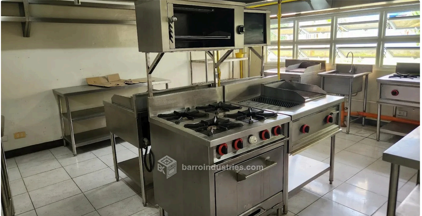
DMMMSU: finished commercial kitchen with range, hood and work tables
